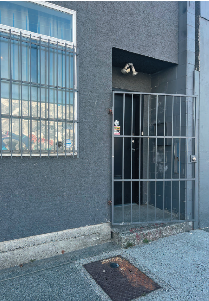
Example of sheltered doorway with security gate, motion lighting and video surveillance signage.
