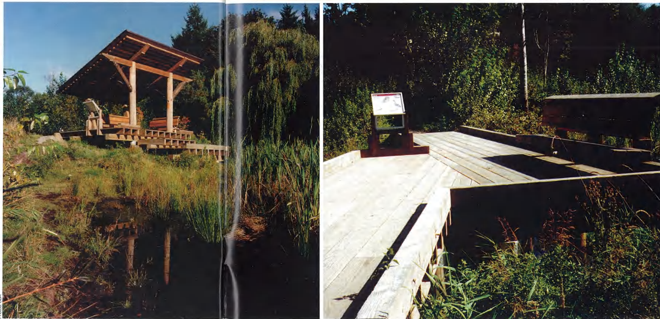
Below: The entry pier is built with timber that was pre-cut and pressure-treated off-site to respect environmental protection measures
