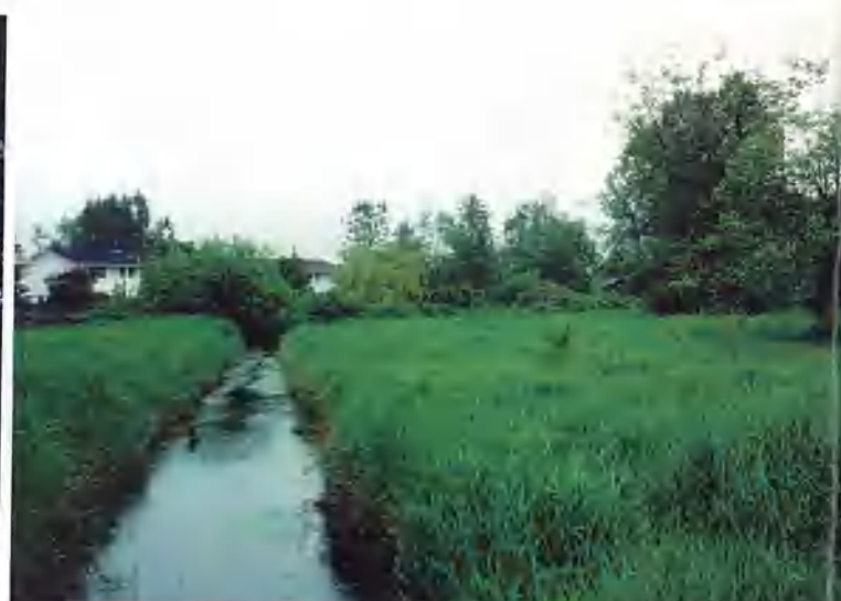
The channelized creek prior to construction. The creek was relocated, deepened and reconfigured.
