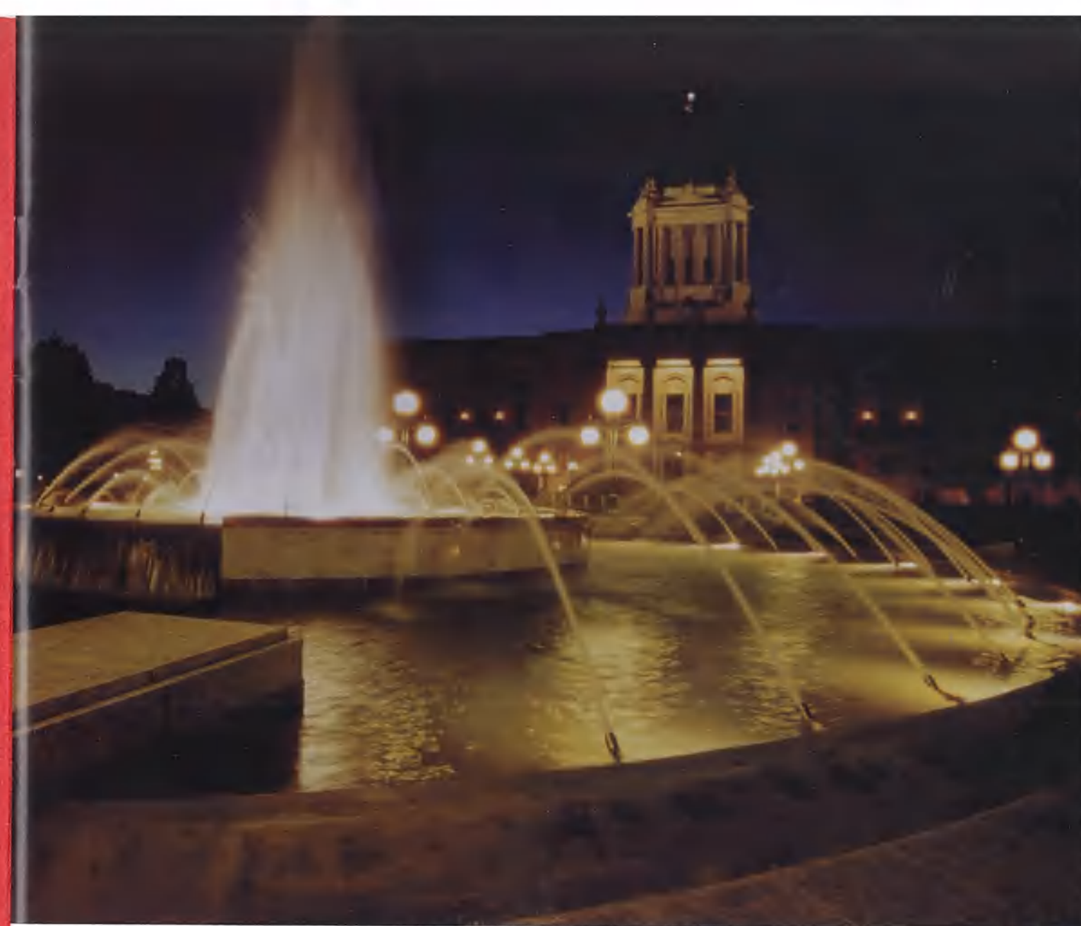
Above: A night view of the Legislative Fountain designed by Gaboury Architects Inc. and UMA Engineering. Wind control devices are included in the design in order to prevent the wetting of the windows of the Legislative Building on windy days.
