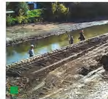
MSE slope construction
